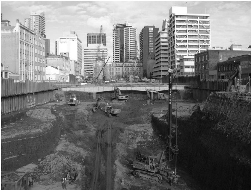
Figure 8 Britomart Station (Eastern end), Auckland under construction in 2002
