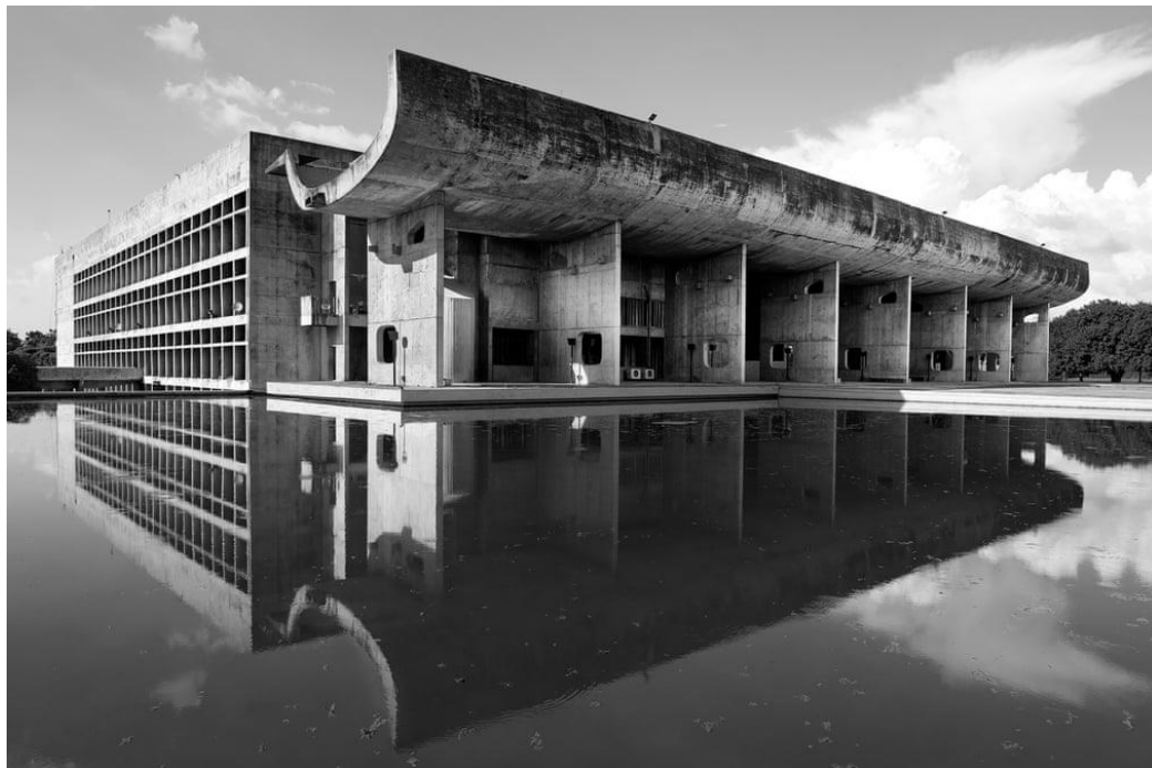
Figure 6 Assembly building, Chandigarh, India
