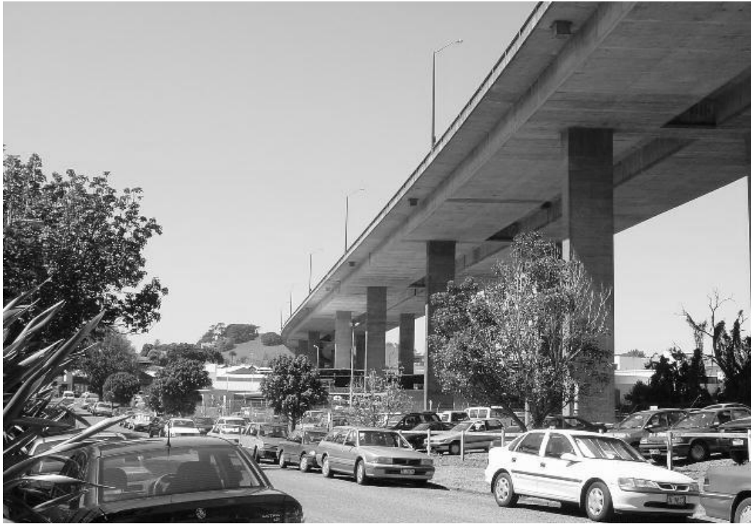
Figure 2 Old Newmarket viaduct on the Southern Motorway, Auckland, New Zealand
